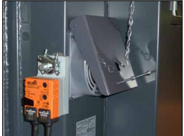
Combustion air inlet for the boiler DCxxGSP closed automatically using Belimo actuator Boiler types DCxxSP(X) from year 2018
