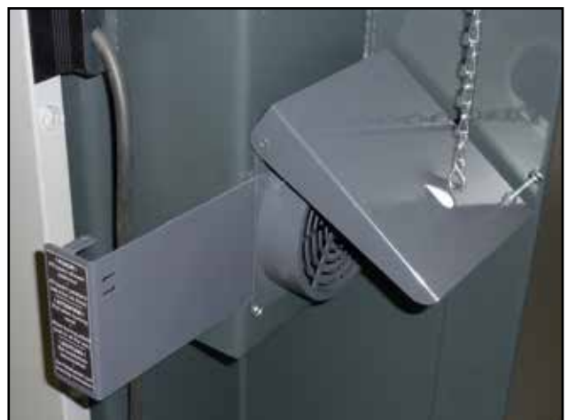
Open valve and regulating flap when burning with manually added fuel
