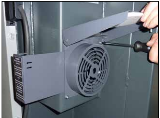
Assembling valve under flap with grille
