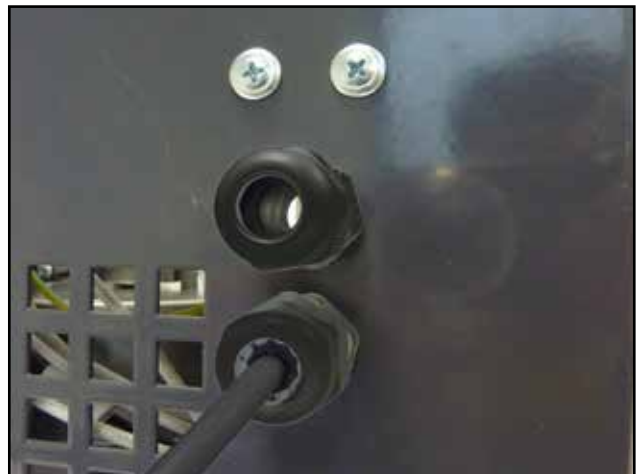
Installation of bushings and cables pulling from the compressor and electrovalve to the burner for DxxPX, PXxx boilers
