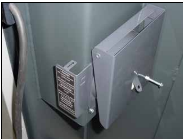
Closed valve and regulating flap when burning pellets
