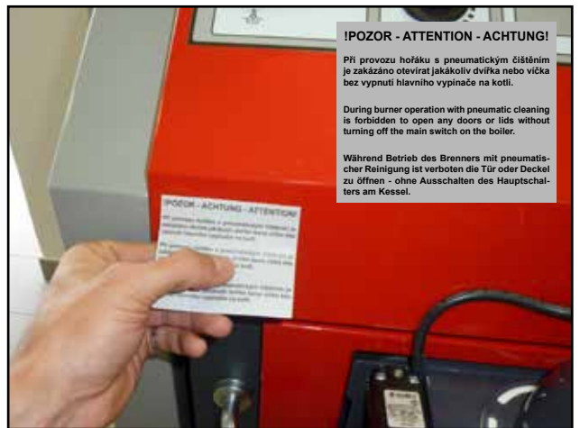
Affixing sticker with important information (ATTENTION – During burner operation with pneumatic cleaning...)
