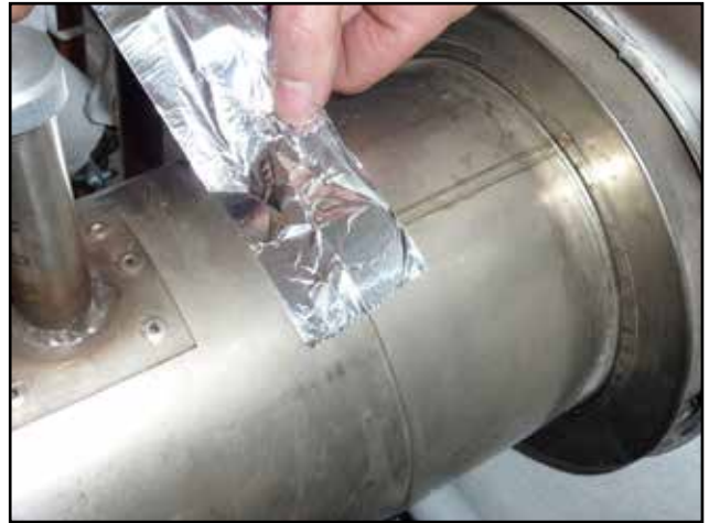
Tightening the flue with an aluminium tape
