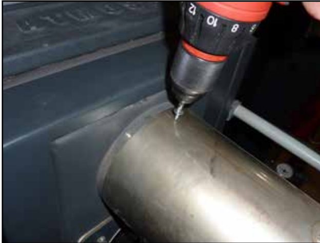
Securing the flue duct with a screw
