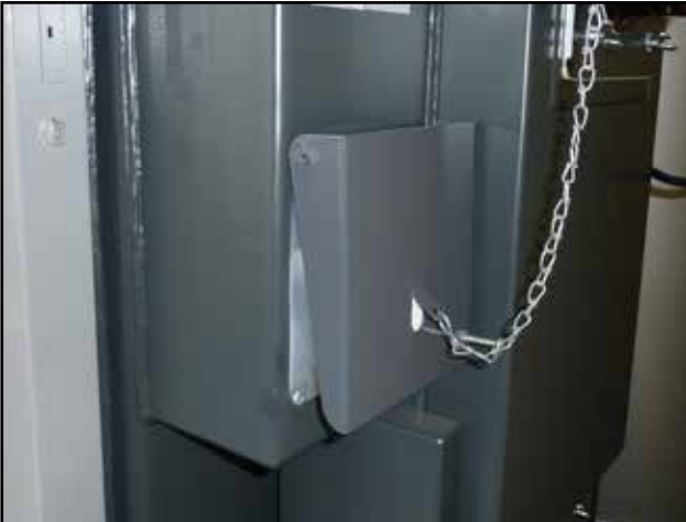
Closed flap for inflow of combustion air for DCxxSP(X), CxxSP, KCxxSP boilers - for models till 2018
