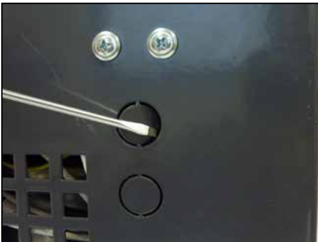
Breaking out holes for bushings on the underside of the burner for DxxPX, PXxx boilers
