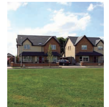
21 of the 5-6 bedroom luxury homes in Straffan Co.Kildare, Ireland. AQUAREA
