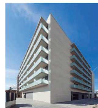
A new building, housing 84 apartments in Cornellà de Llobregat, Barcelona. AQUAREA
