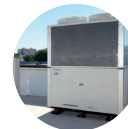
2012 New GHP units. Panasonic's gas-driven VRF systems are ideal for projects where power restrictions apply.
