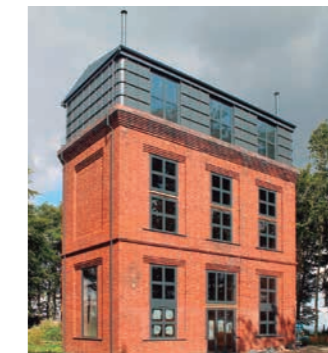
An water tower has been converted into a stunning family home. Yorkshire, UK. AQUAREA
