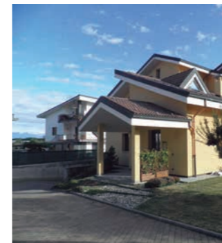
Duplex in Boves, CN. Italy. AQUAREA
